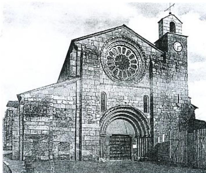
Abb. 102a Santa Maria in Meira, Fassade
